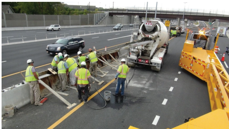
Figure 5. A Work Zone Protected by MBT (40)
